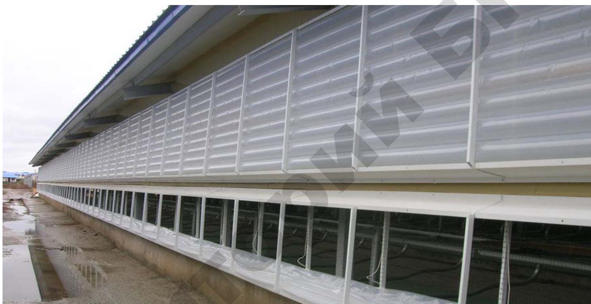
Figure 4.10. Special membranes' usage instead of ordinary curtains in the cattle keeping premises
