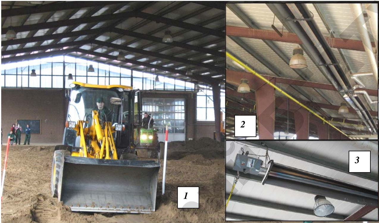
Figure 3.12. The gas infrared heaters' usage in covered pavilions: 1 – a general view of a pavilion; 2 – heaters' placement along the longitudinal wall, where training working places (desks) are found; 3 – a general view of a gas heater
