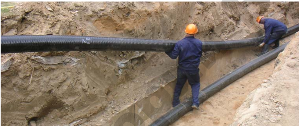
Figure 5.4. Flexible pipes laying “Kasaflexx”
