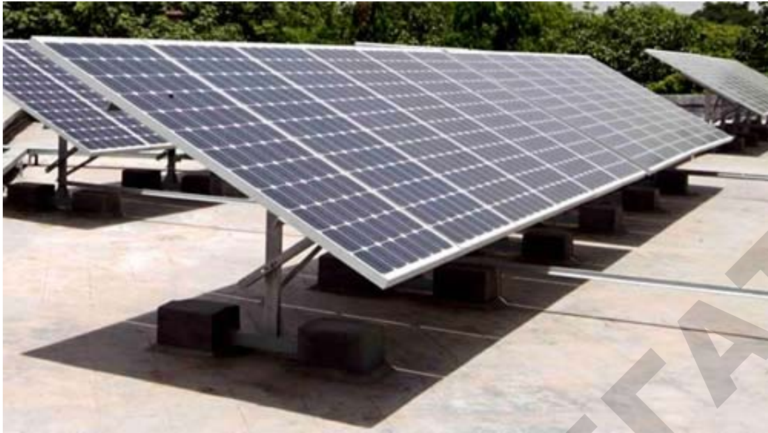
Figure 7.3. A general view of solar photovoltaic panels
