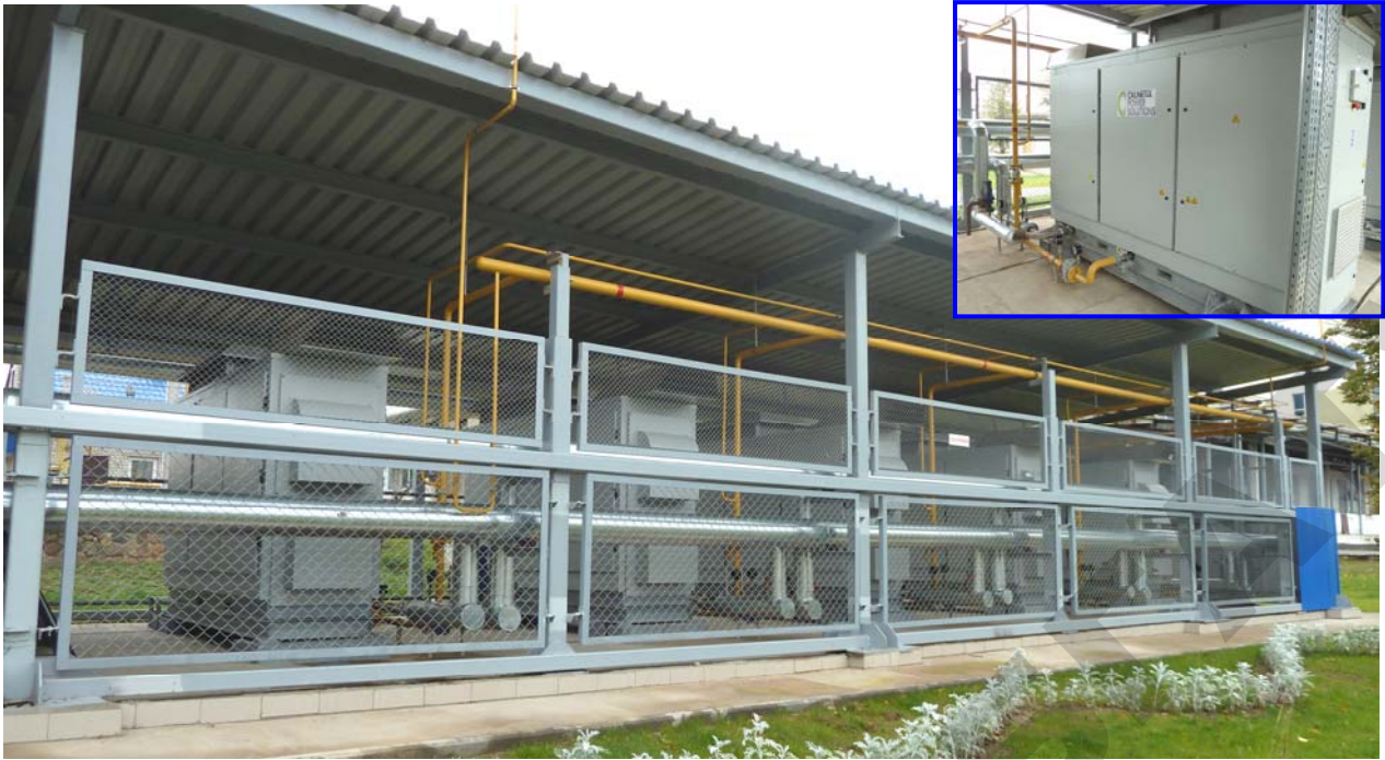
Figure 6.12. Block of microturbine installations at OJSC “Glubokoe dairy-canning factory”, Vitebsk region
