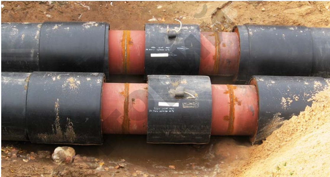
Figure 5.2. Placement of PI-pipes in the channel (without pipe-couplings)
