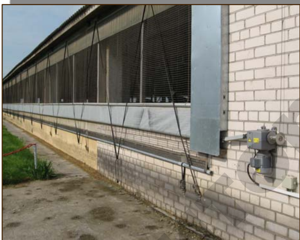
Figure 4.9. Natural ventilation through an air curtain
